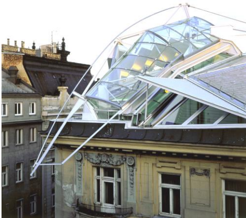
Rooftop Remodeling Falkestrasse Coop Himmelb(l)au,
